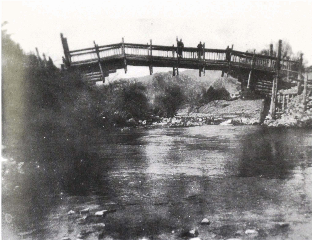
The typical cantilever bridge over the Hsia-ho River in front of the Bla-bran Monastery.
